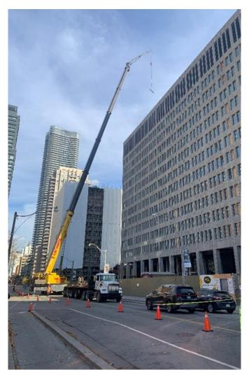
In November, a portion of Wellesley Street West was closed to enable the safe operation of a mobile crane to lift steel onto the roof of the Ferguson tower.
